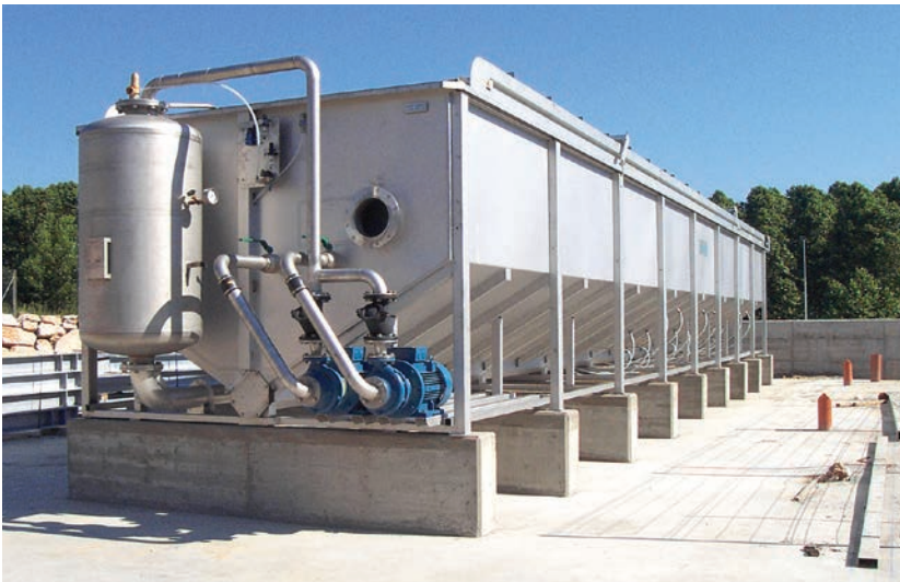
Top of Page: several stages of water treatment Above: water, mankind´s most precious resource Upper Left: surface aeration basin Lower Left: dissolved air floatation unit Opposite Page: baby chicks are fed from the very moment they arrive in the farm
