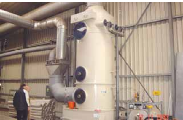
Figure 3: A chemical scrubber (Courtesy: Reinluft)
