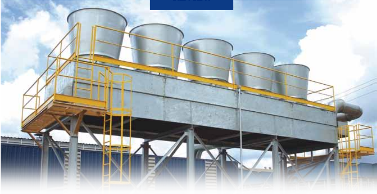
Fig. 2: Air cooled condensers in a rendering plant
